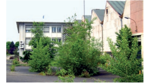
Usine Schindler Illzach © Yvan Renckly
